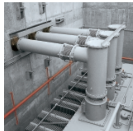
Fig. 55: Transformer termination modules
