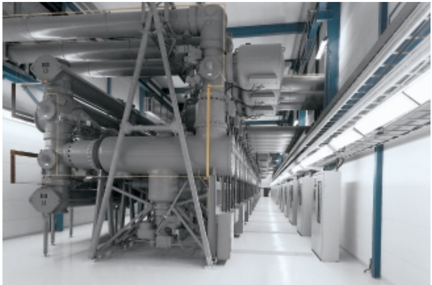
Fig. 47: 8DQ1 switchgear for rated voltage 420 kV
