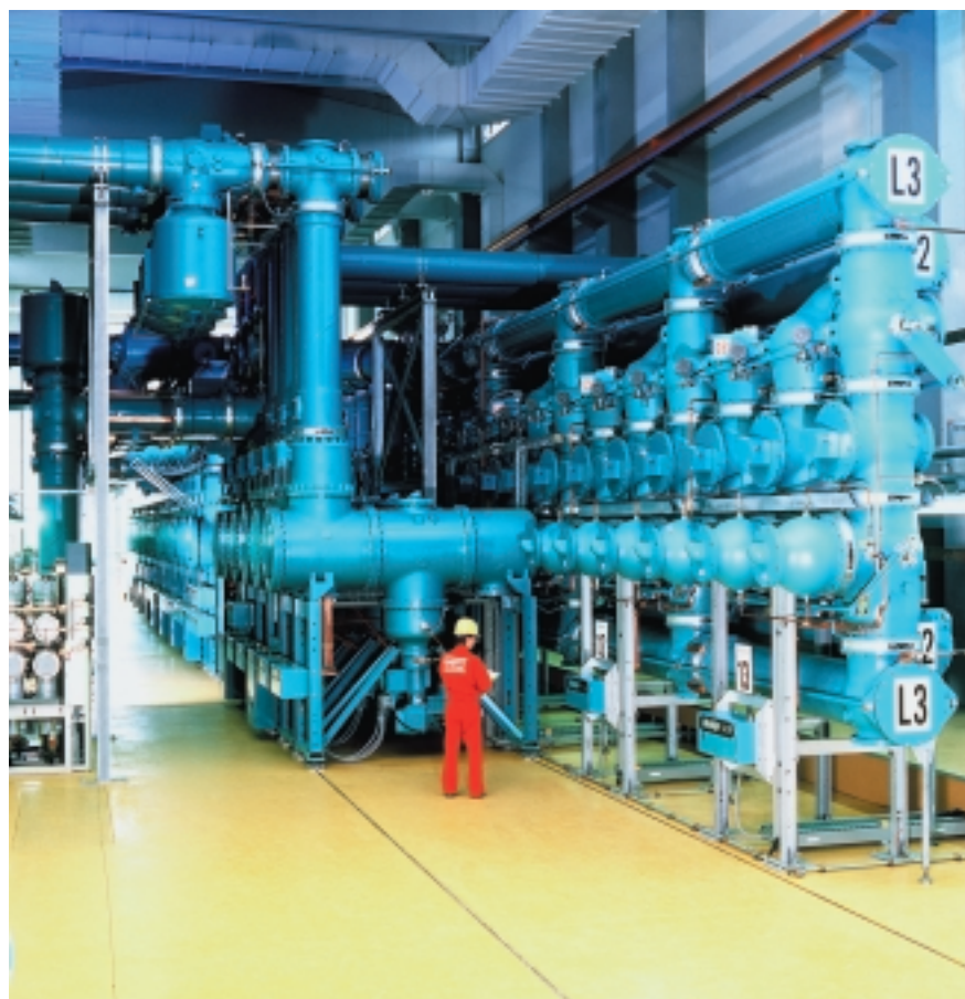
Fig. 56: The modular system of the 8DQ1 switchgear enables all conceivable customer requirements to be met with just a small number of components
