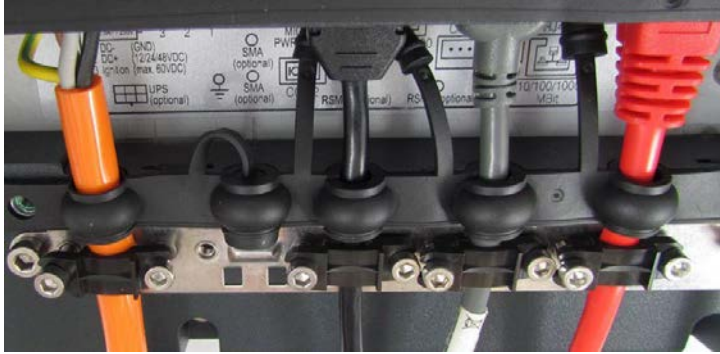
Fig. 8.8: Unused cable outlets sealed off with blind plugs
