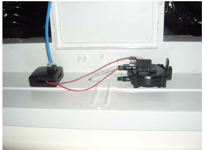
FIG 2. RETURN AIR AND ROOF AIR INSTALLATION OF ENTHALPY SENSOR AND PRESSURE SENSOR IN GRILLE
