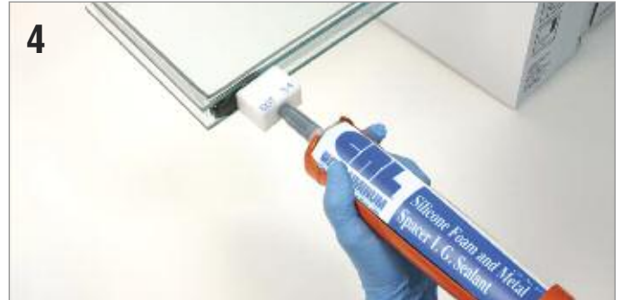
Apply CRL Hot Melt Butyl or Cat. No. 877 Sealant to seal the unit.
