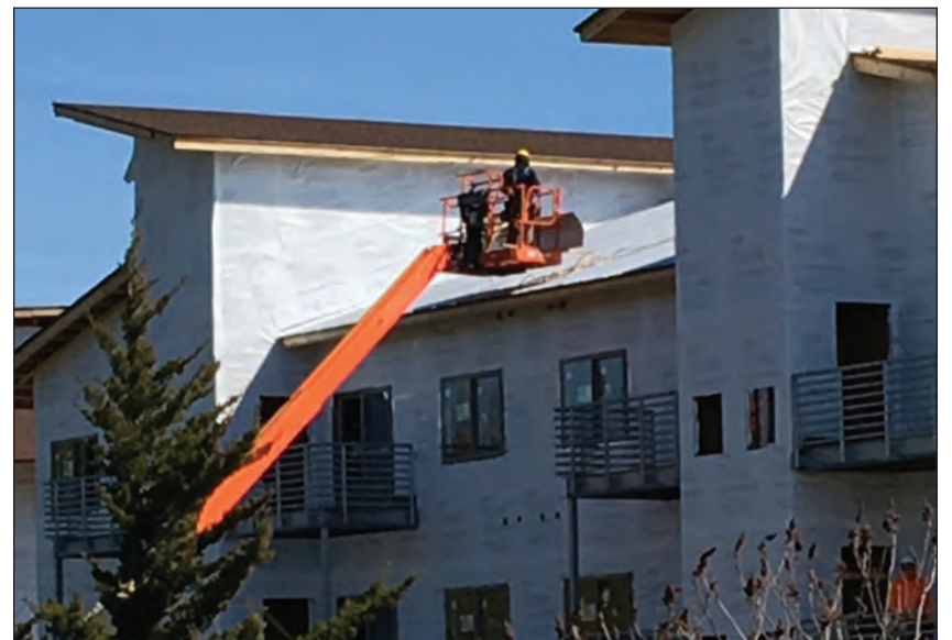
Construction restarts for Forsberg Real Estate Company at Elevation Apartments in Okemos.
