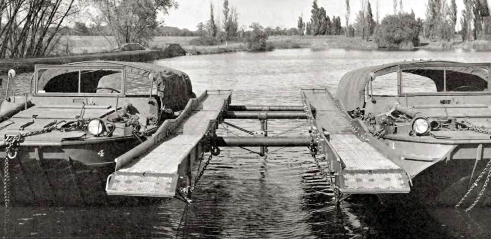
Above: This was described as a 'teeter type dry ferry' and used a pair of DUKWs tied together with cross tubes.
