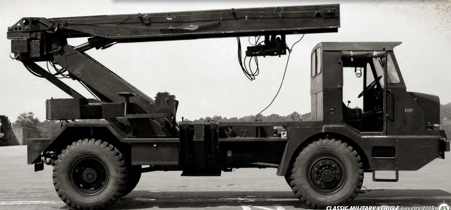
Below: Nubian 4x4 chassis with Bedford RL engine and running gear, used to provide the basis for a missile-handling crane. Registered 00EX21, the vehicle was one of two delivered in 1965 to the School of Artillery.
