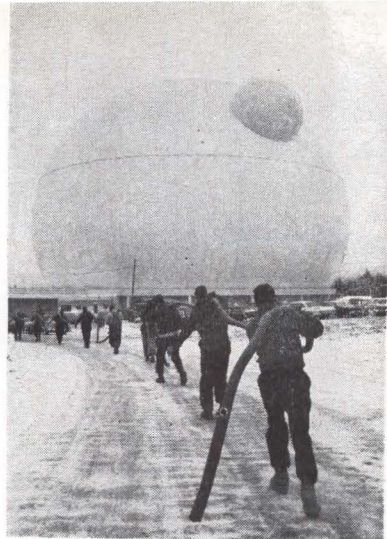
Antennas at main ground station at Andover were erected this winter under a huge inflated dome
