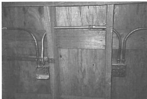
Two Gang Boxes Daisy-Chained Together
