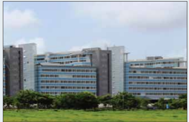
The world's largest diamond exchange, Bharat Diamond Bourse, spread across 20 acres, is secured by Siemens' integrated security solutions.
