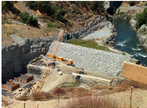
Folsom Dam Auxiliary Spillway Phase IV - JV (CA) Construction phase services support for spillway control structure
