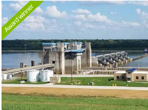
Olmsted Dam Construction - JV (IL) Used innovative "in-the-wet" methods to deliver one of the largest U.S. civil works projects to improve critical inland marine infrastructure
