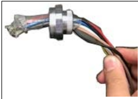
Figure 9: Fixing Union to Conduit
