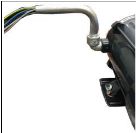
Figure 20: Moving the Conduit
