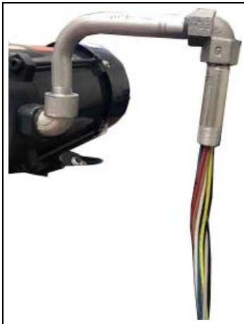
Figure 22: Tightening the Conduit
