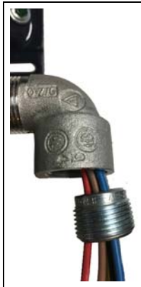
Figure 5: Bushing inside the Elbow Joint
