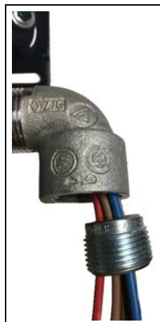
Figure 18: Routing Wires through Bushing
