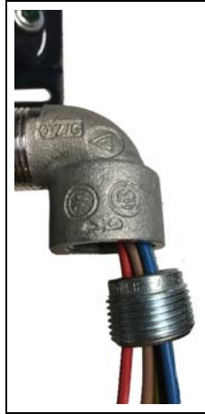
Figure 27: Routing Wires through Bushing
