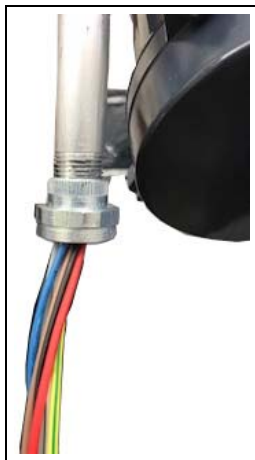
Figure 9: Fixing Union to Conduit
