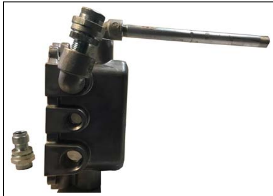
Figure 60: Inserting Grade 2 Conduit
