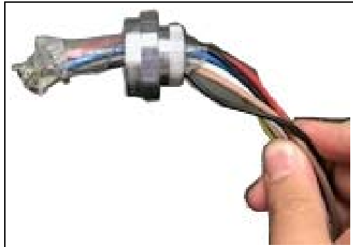
Figure 24: Fixing the Union to the Conduit
