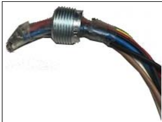
Figure 11: Routing Wires through Bushing
