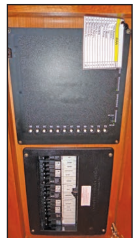
Figure 9-1: Circuit breaker box
