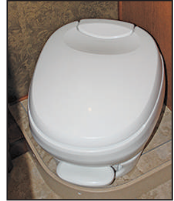
Figure 13-10: Toilet pedal flush lever
