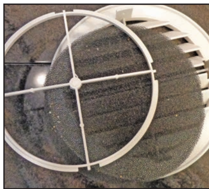
Figure 3-3: Round vent filter
