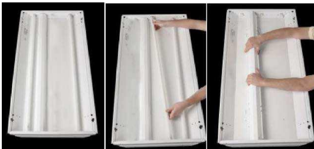
a) Troffer et lampes b) Retirer les lampes fluorescentes c) Remove ballast cover (lens removed)
