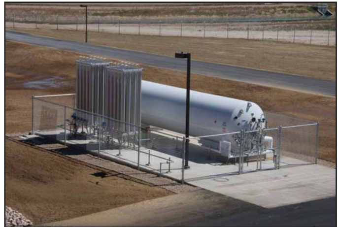
System installation at site
