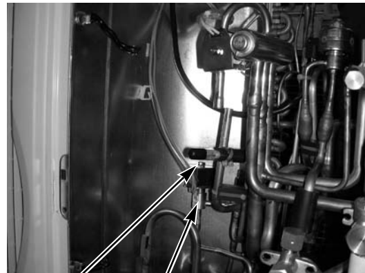
Bypass valve fixing screw
