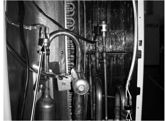
High pressure switch (63H)
