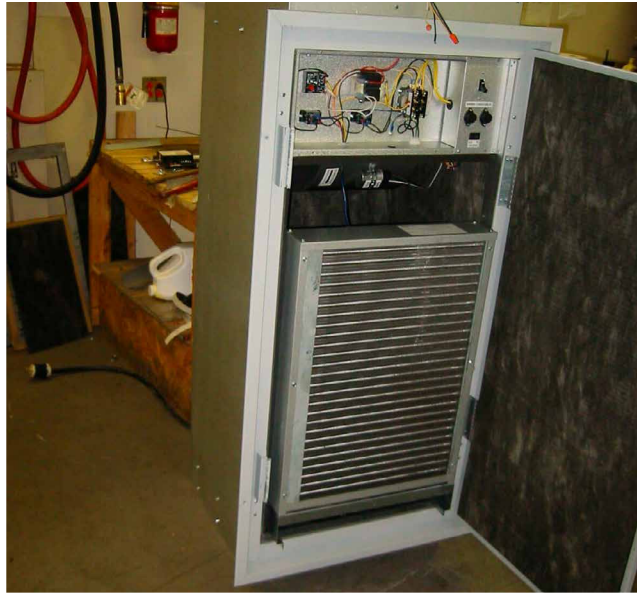
Figure 29: Check the chassis alignment
