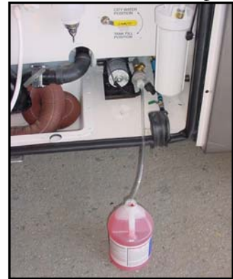
Figure 14-15. Winterizing Process
