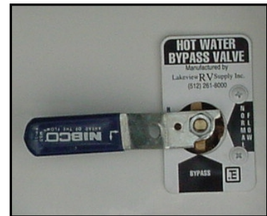
Figure 11-7. Water Heater Bypass Valve
