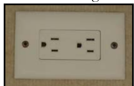
Figure 7-5. 120 VAC Receptacle
