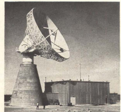
60-FOOT ANTENNA provides pencil beam for tracking reentering missiles
