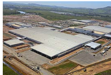
The new Resende Plant, to be surrounded by a "Green Belt" that helps absorb CO 2 and reduces noise levels.
