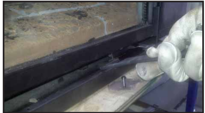
Figure 11.2. Glass Clip Tool Location
