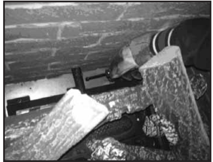
Figure 1. Air Shutter Location
