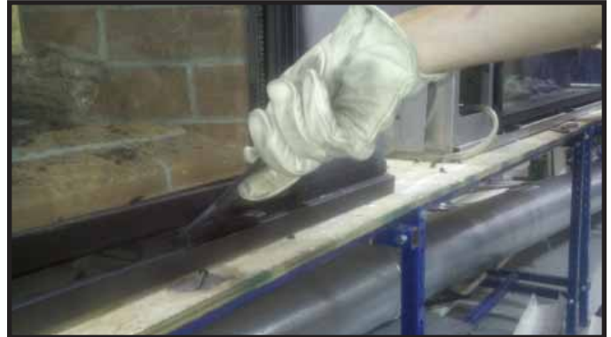
Figure 11.3. Inserting Glass Clip Tool
