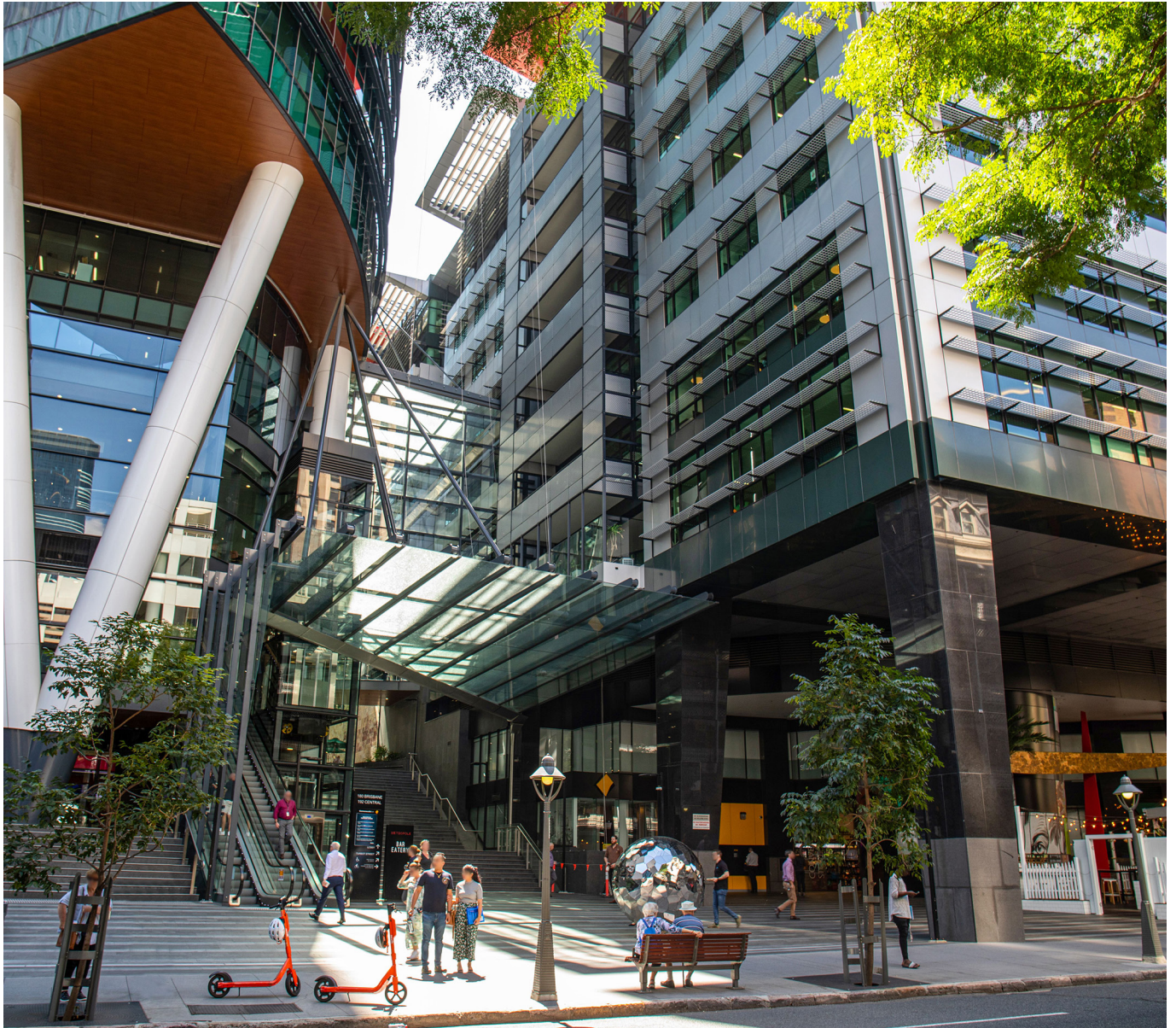
Figure 3: Daisho/Mincon Building at 190 Ann Street
