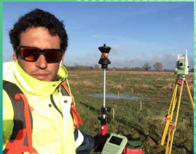
Staking out a photovoltaic park in Lyon, France
