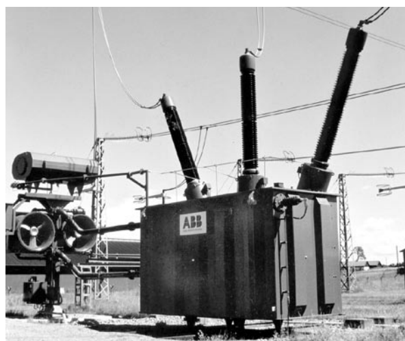
Shunt reactor, 420 kV, 150 Mvar
