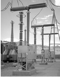
Circuit breaker HPL 550B2 controlled by Switchsync™ for smooth shunt reactor switching.
