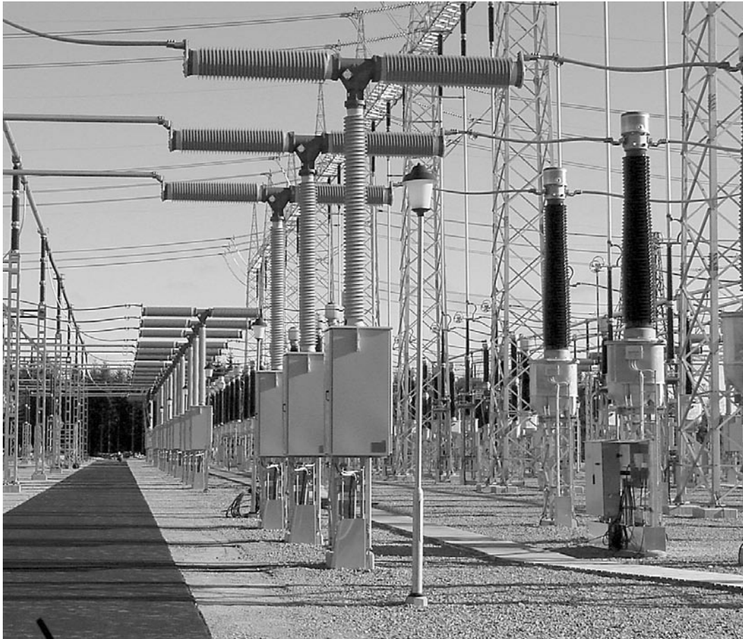
Disconnecting circuit breaker for controlled power transformer switching in a 420 kV substation
