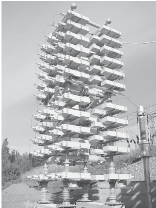
One phase of 300 kV, 200 Mvar capacitor bank, Norway
