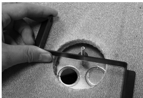
2 Attach the Z bracket to the ceiling tile and the back plate.
