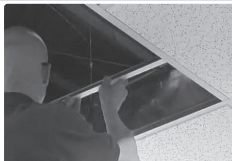
2a Place the T-rails on the T-frame.
