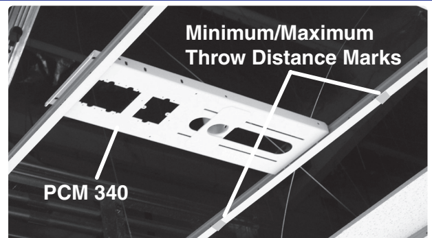
2b Place the PCM 340 on the T-bar
