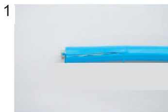
1 Expose inner vinyl sheath.
