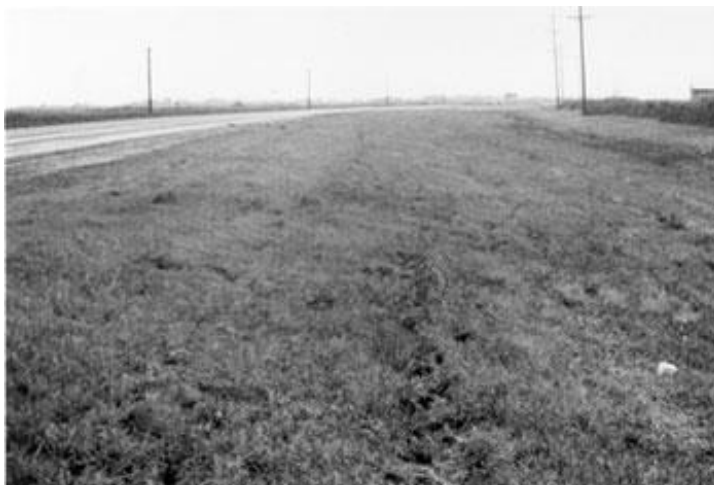
Figure A-1: Typical Roadway with Roadside Hazard Rating Equal to 1
