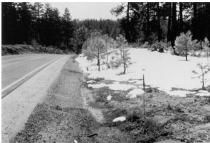
Figure A-3: Typical Roadway with Roadside Hazard Rating Equal to 3
