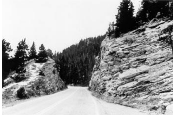
Figure A-7: Roadway with Roadside Hazard Rating Equal to 7
