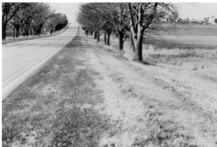
Figure A-5: Typical Roadway with Roadside Hazard Rating Equal to 5
