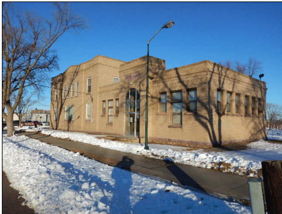
SOUTHEAST CORNER - FRONT VIEW
