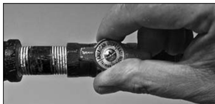
Figure 30: Gas valve in "on" position
