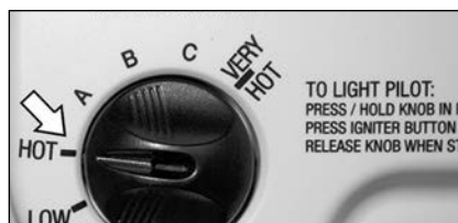
Figure 34: Adjust the gas control knob to "HOT".
