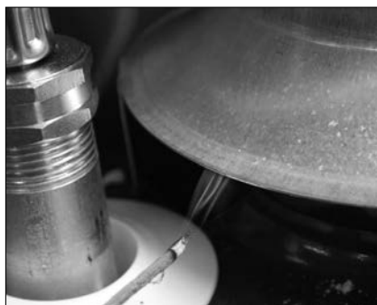
Figure 33: Test the air supply and vent to make sure the water heater has adequate air and is venting properly.
