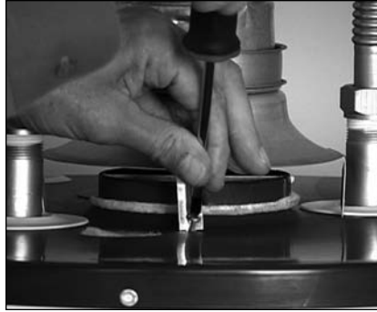
Figure 24: Install the new draft hood and secure with screws.
