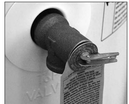
Figure 18: Temperature and Pressure Relief Valve
