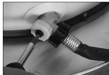
Figure 12: Draining the old water heater.
