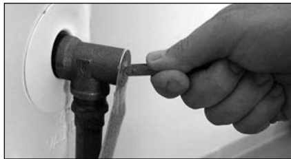
Figure 41: T&P Relief Valve.
