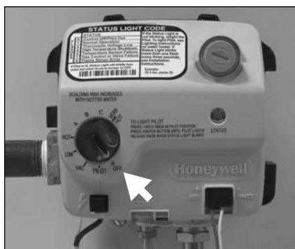
Figure 43: Gas control/valve.
