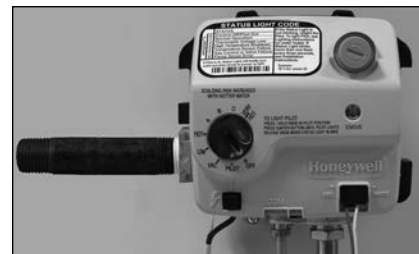
Figure 47: Gas control/valve with threaded pipe.
