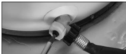
Figure 38: Draining the water heater.
