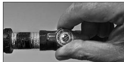
Figure 48: Gas valve in "on" position.
