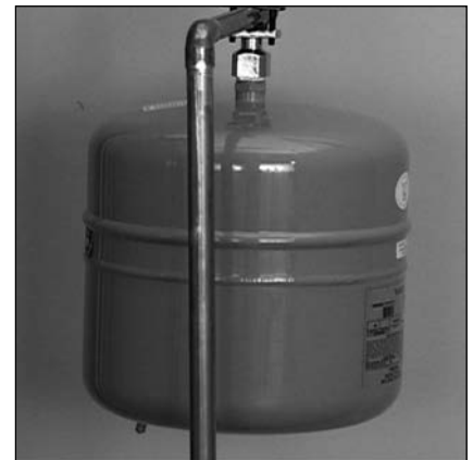
Figure 23: The Thermal Expansion Tank should be pressurized with air, using a hand pump, to match the home's incoming water pressure.
