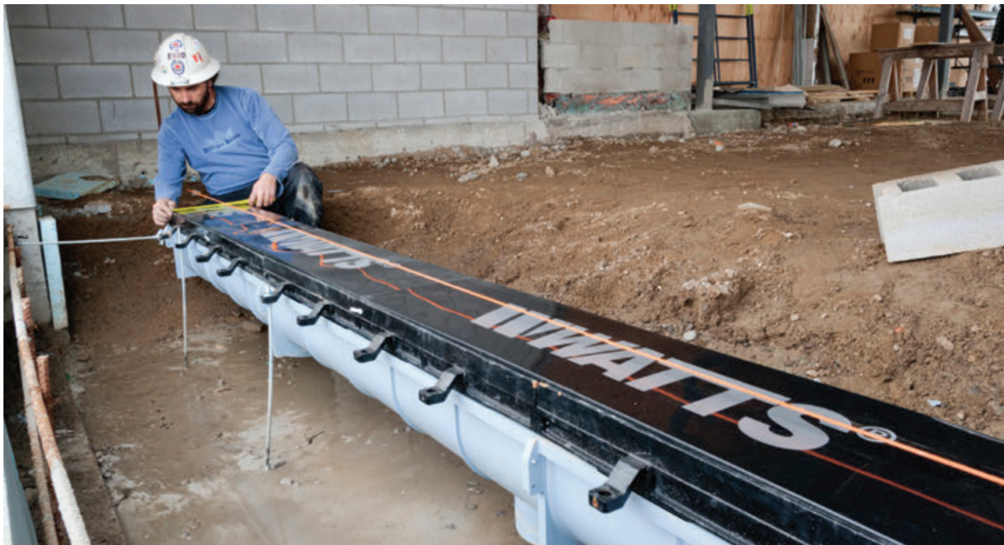
A Watts Dead Level® trench drain installation.
