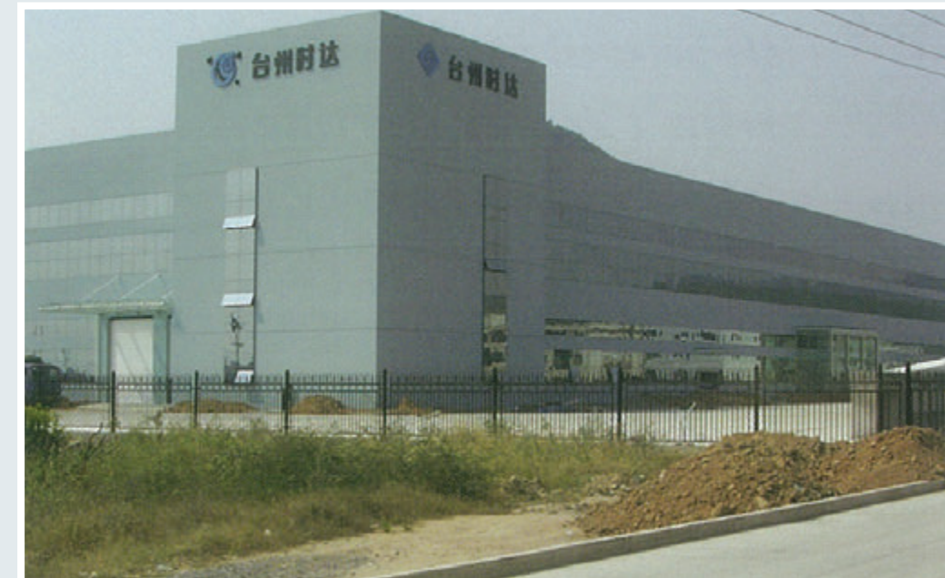
Watts' Taizhou Shida Pipe Product Manufacturing Co., Ltd., formerly called Chen Guan Metal Hose Factory.
