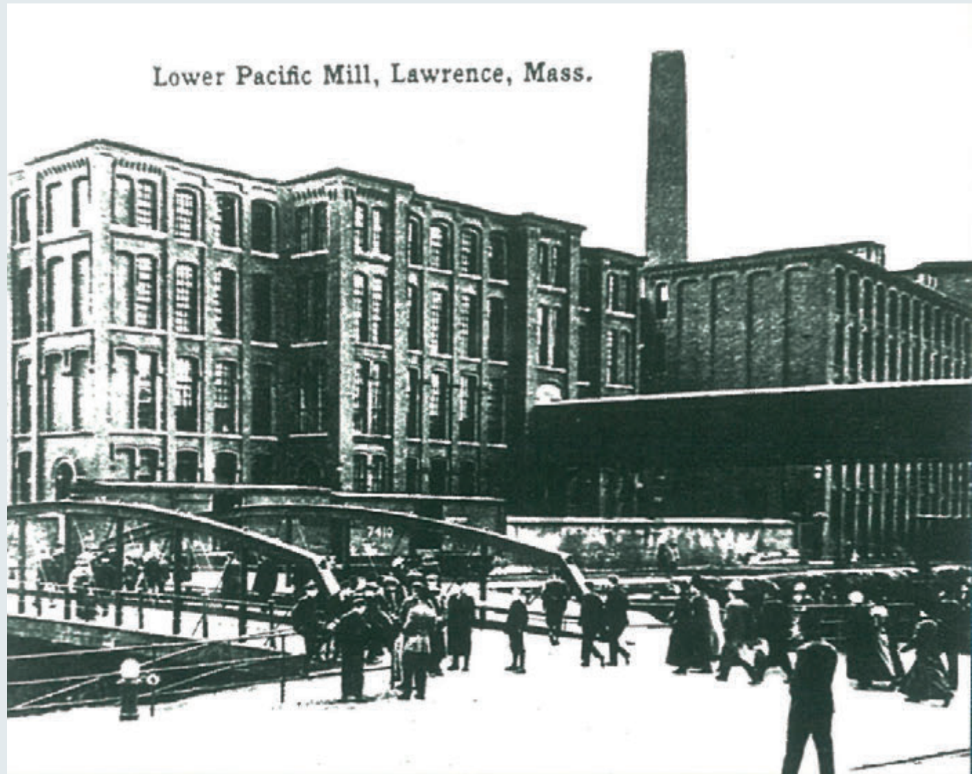
Joseph E. Watts chose the Pacific Mills in which to work in 1857. It was common practice in the 19th century to recruit skilled workers from England because many of the leading engineers in the textiles and waterworks industries were themselves English immigrants.
