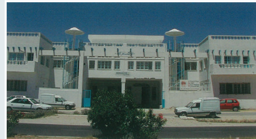
ADEV's (now Watts Electronics) manufacturing plant in Monastir, Tunisia, provides Watts with cost-effective production of HVAC electronic heating-control thermostats.
