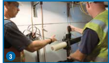
3 Remove the semi-conductive shield...
