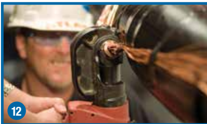
12 Connect neutral wires as required.
