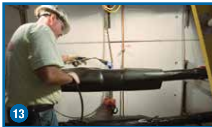
13 Position and shrink cover-ups.
