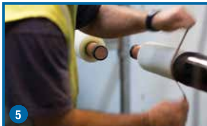
5 Sand semi-conductive shield to provide a smooth transition to the cable insulation.
