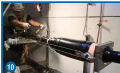
10 Reposition the assembly tool and pull the TCJ joint housing into the final position on the cable.
