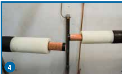
4 ...and bare the conductor.
