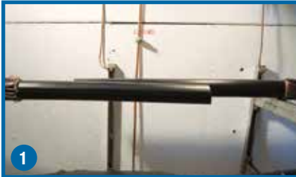
1 Overlap cables, straighten and strip back jacket.
