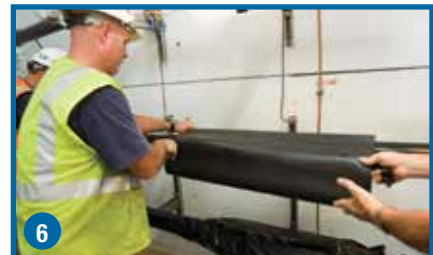
6 Store the cover-up sleeve on each cable.
