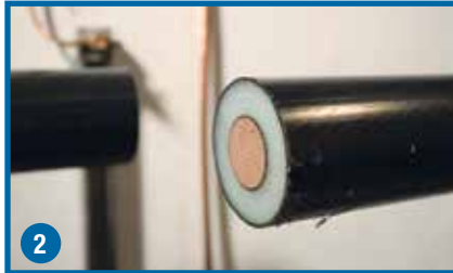
2 Square cut the cable at the center line of the joint.
