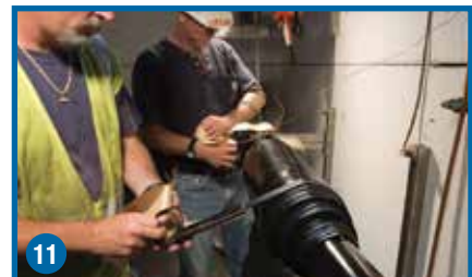
11 Seal joint ends with mastic wrap.
