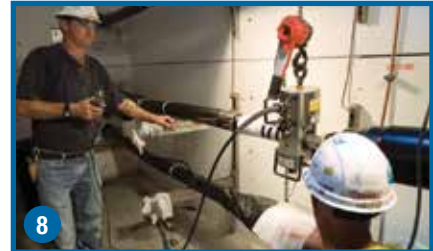
8 Join the conductor using a compression, welded or other type of connector.
