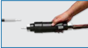
Place Elastimold® Shrink-Fit Joint in position.
