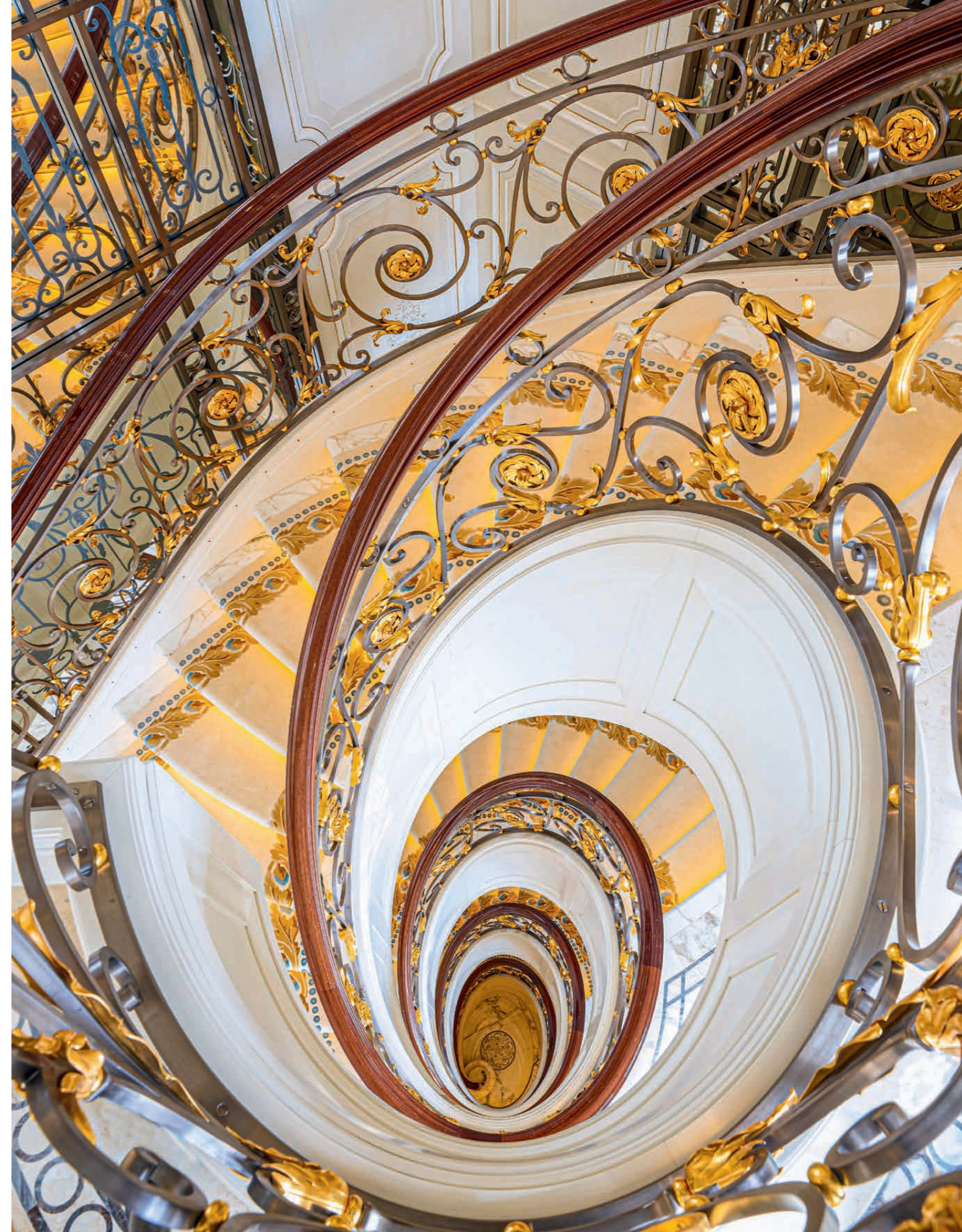
Deliberate copy: for the spiral staircase the owner dispatched Andrew Winch's team to the Hotel Le Bristol in Paris. The outcome of their efforts includes true-to-original handrails as well as wrought-iron balustrades with auricular-style motifs and gilded acanthus leaves.
