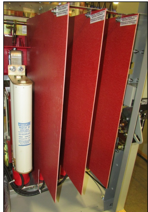
Fig. 45 Fuse Barrier Placement
