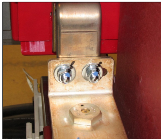
Fig. 42 Check Electrical Joints
