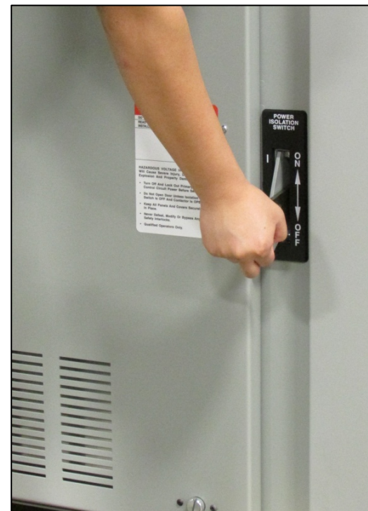
Fig. 39 Closing Isolation Switch
