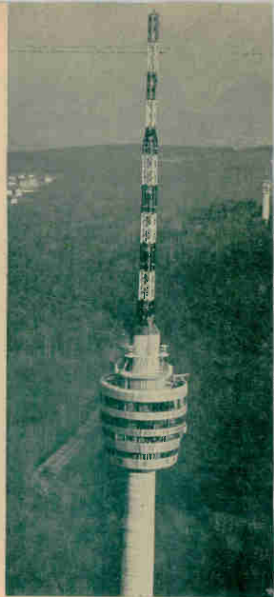
Television tower just outside Stuttgart. The five-ringed structure below the antenna is a restaurant; in some German installations they slowly rotate around the concrete support
