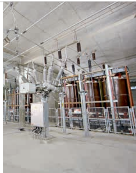
5b Appareillage hybride SF 6 /air PASS M00 72,5 kV
