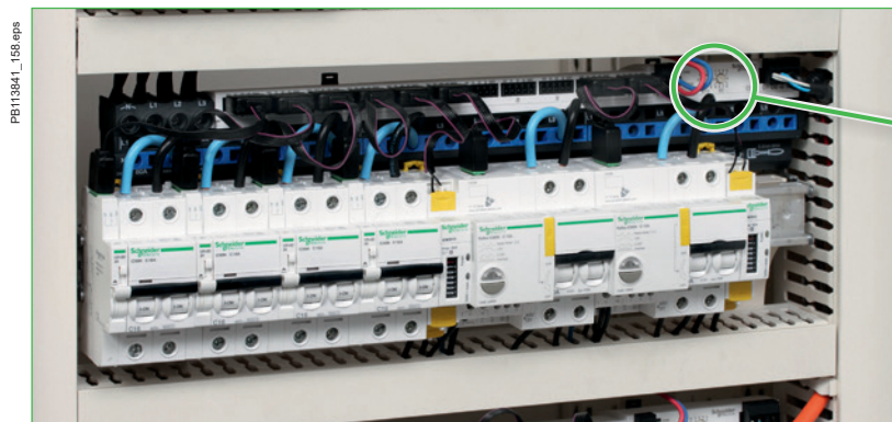
Rotary Switch Modbus addressing
