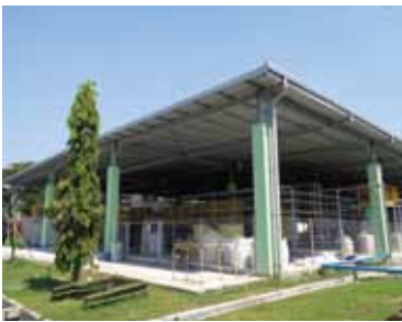
Wastewater treatment facility in Indonesia
