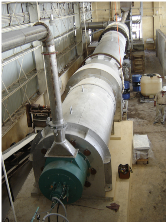
Salt Dryer with Vortometric installation
