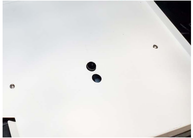
Install supplied 1.0625 dome plugs into holes in floor. It is recommended to also use silicone to prevent leaks.
