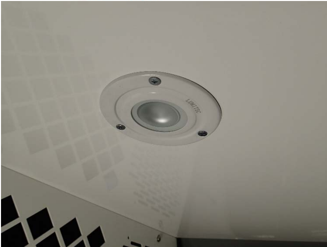
Install LED dome light with hardware included as per instructions in the dome light kit.
