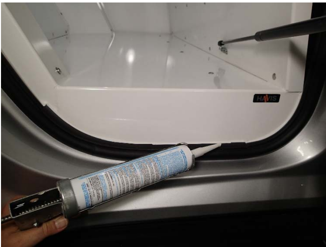
Neatly silicone / caulk the lower seams to shed water out of vehicle. Note: The floor is designed to minimize the need for sealant. Caulk (sealant) is mostly needed where the floor meets the doorsill and lower filler panels.
