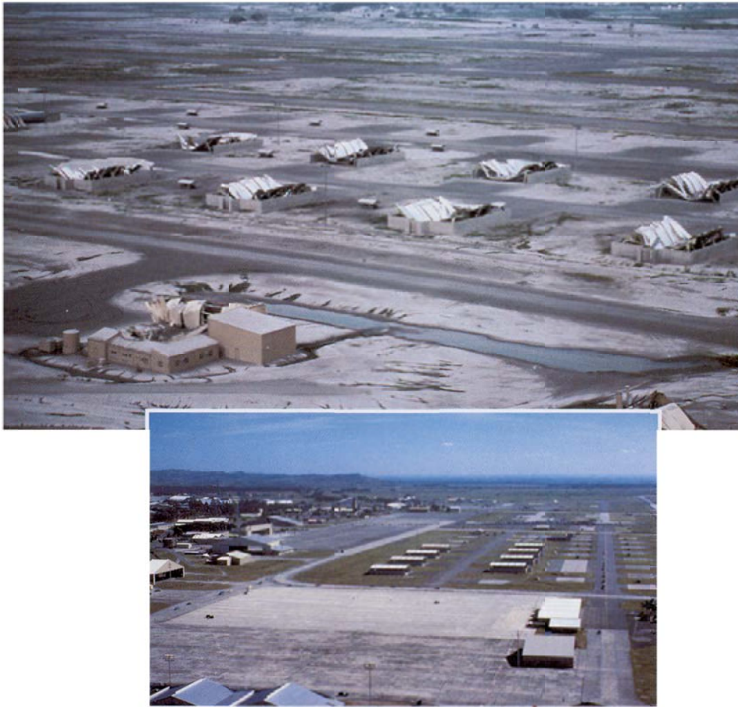
Figure I-5-1. Hangars at Clark Air Force Base, Philippines, before — see insert photo (10 June 1991) — and after (24 June 1991) major eruption on 15 June, 1991. (from Casadewall)
