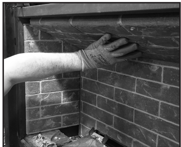
Figure 11.6 Install Right Refractory Panel
