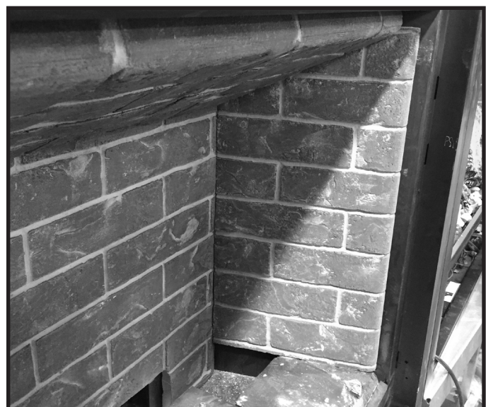
Figure 11.7 Right Refractory Panel Installed
