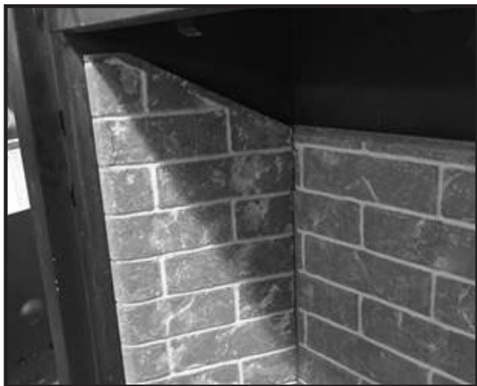
Figure 11.4 Install Left Refractory Panel
