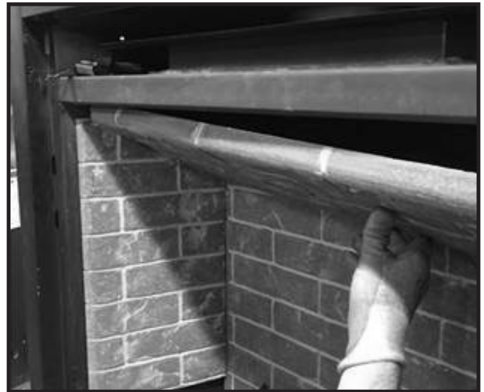
Figure 11.5 Install Top Refractory Panel
