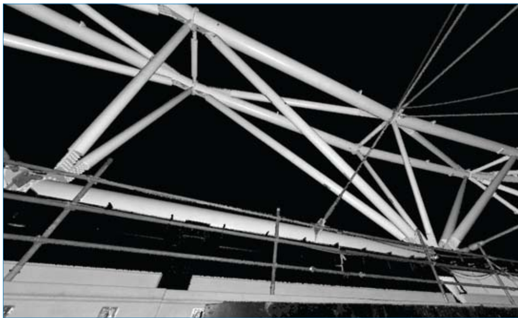
This high-resolution scan of the roof-supporting structure was taken using a high-speed phase-based 3D laser scanner. The point cloud is displayed in grey-scale intensity mapping, with locating holes and individual rivets visible.
