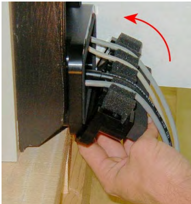
Figure 9-4. Installing Lower Flange
