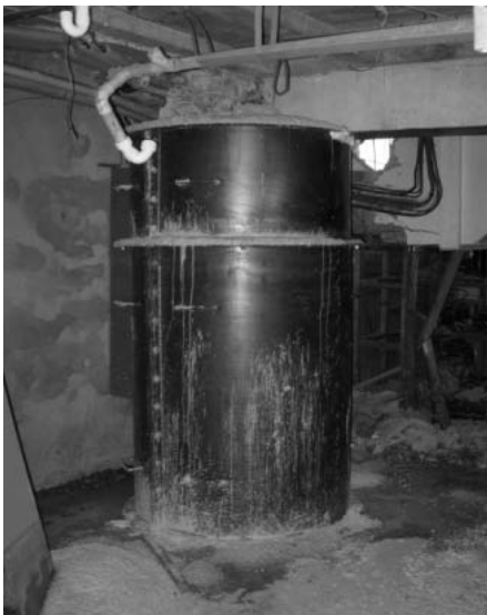
Damaged columns with completed encasement
