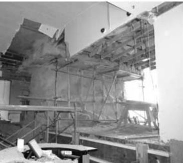
Overall View of Repair Using Shotcrete
