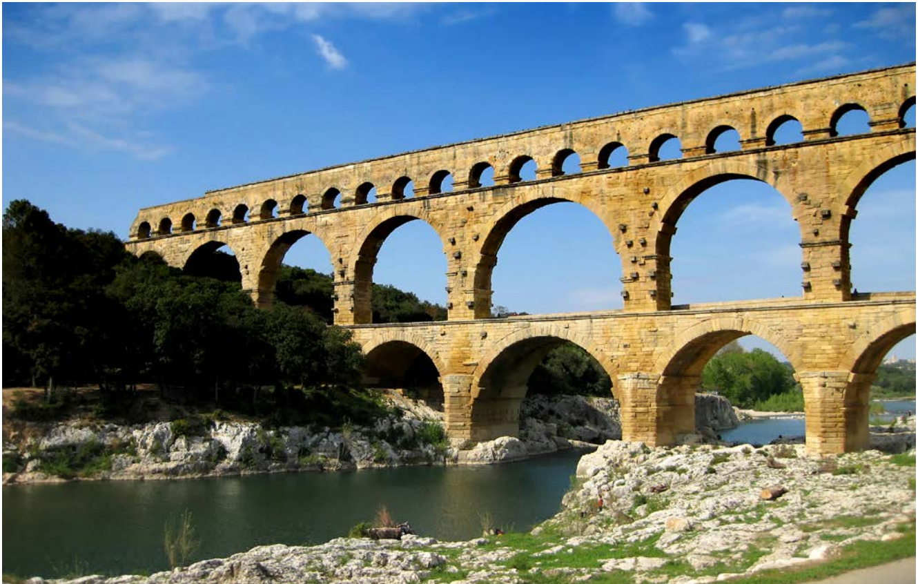
Roman aqueduct, the Pont du Gard, near Nimes, France
