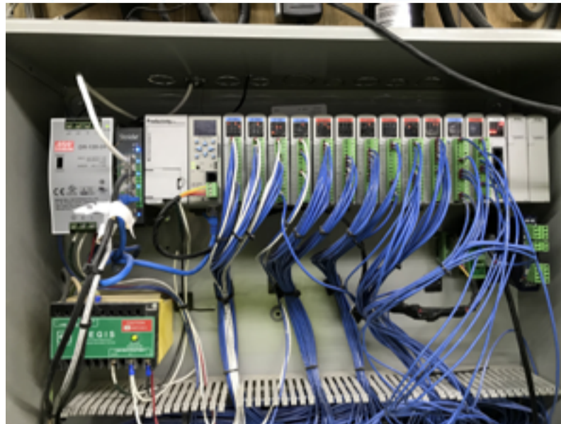
Figure 4: Productivity2000 Control System CTC Crushing's electrician installed and wired the Productivity2000 controller in 15-slot racks to handle the high I/O count.
