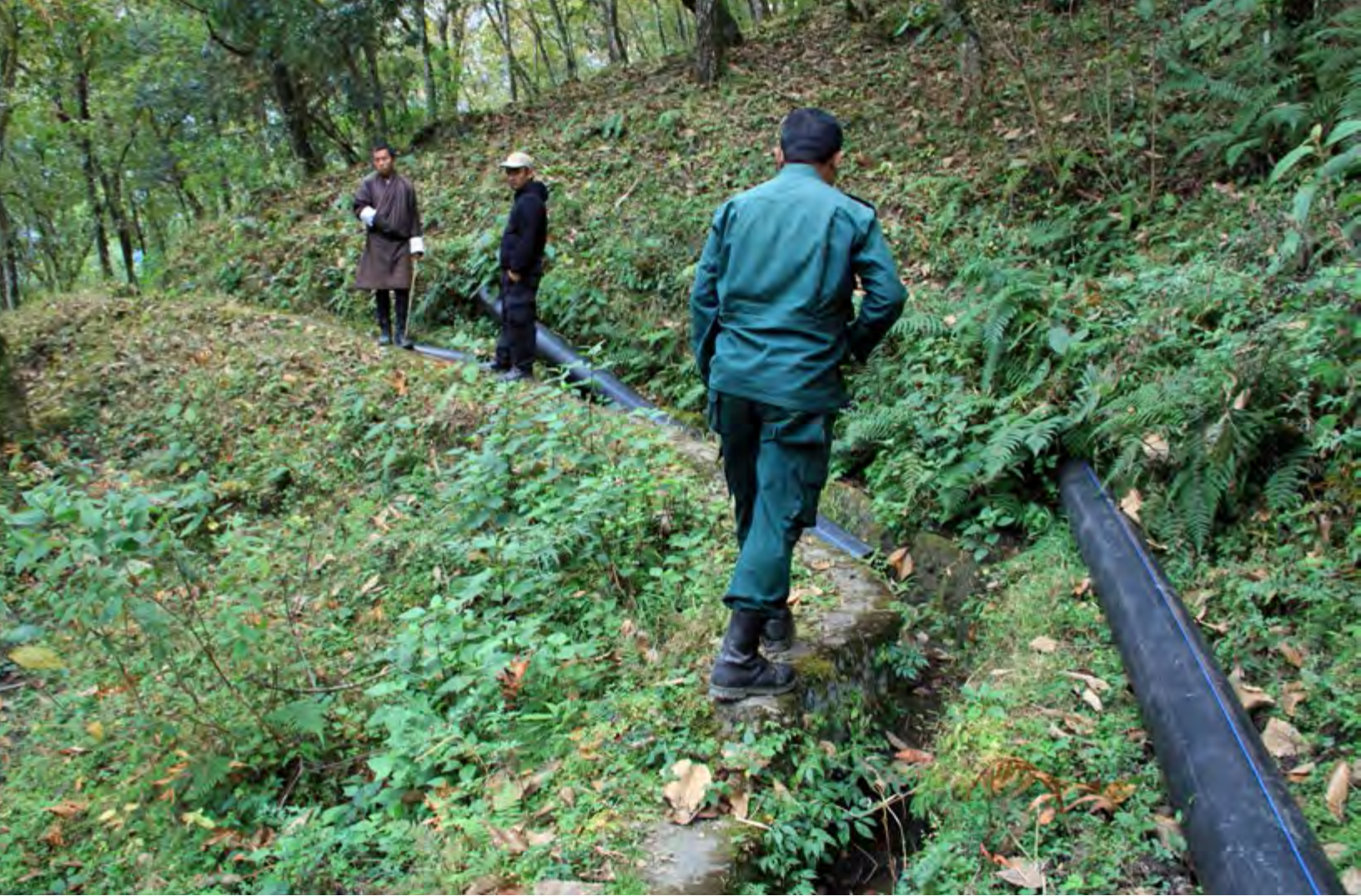
An old village irrigation canal in the process of being replaced with a water-efficient irrigation pipe, Gangzur Geog, Wangchuck Centennial National Park, Bhutan. © WWF Bhutan
