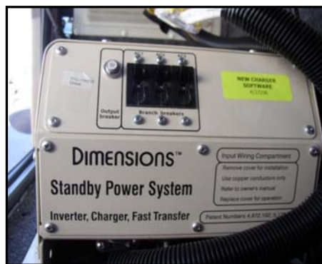
Figure 7-13. Inverter/Converter
