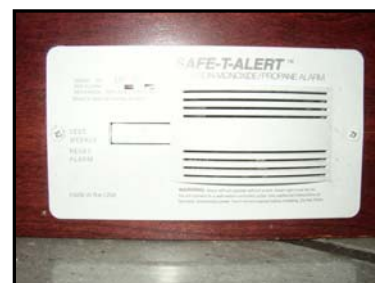
Figure 3-6. CO/LP Gas Detector
