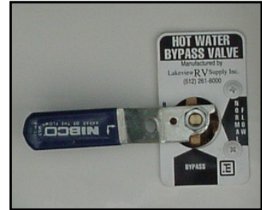
Figure 11-11. Water Heater Bypass
