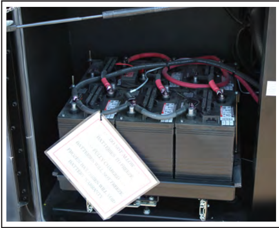
Figure 10-4: House batteries
