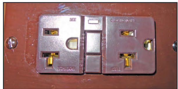
Figure 10-13: GFCI receptacle
