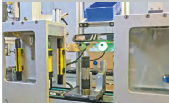
For the safe assembly of roller shutter motors, Elero relies on the EZ Screen safety light curtains and a pick-to-light solution from the Turck range. Page 30
