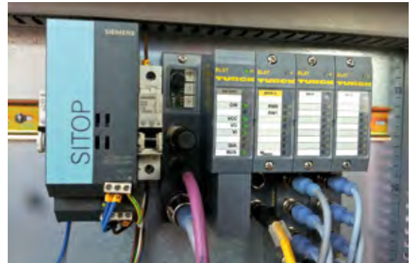
In addition to the RFID read-write heads also switching signals are connected via the BL67 system
