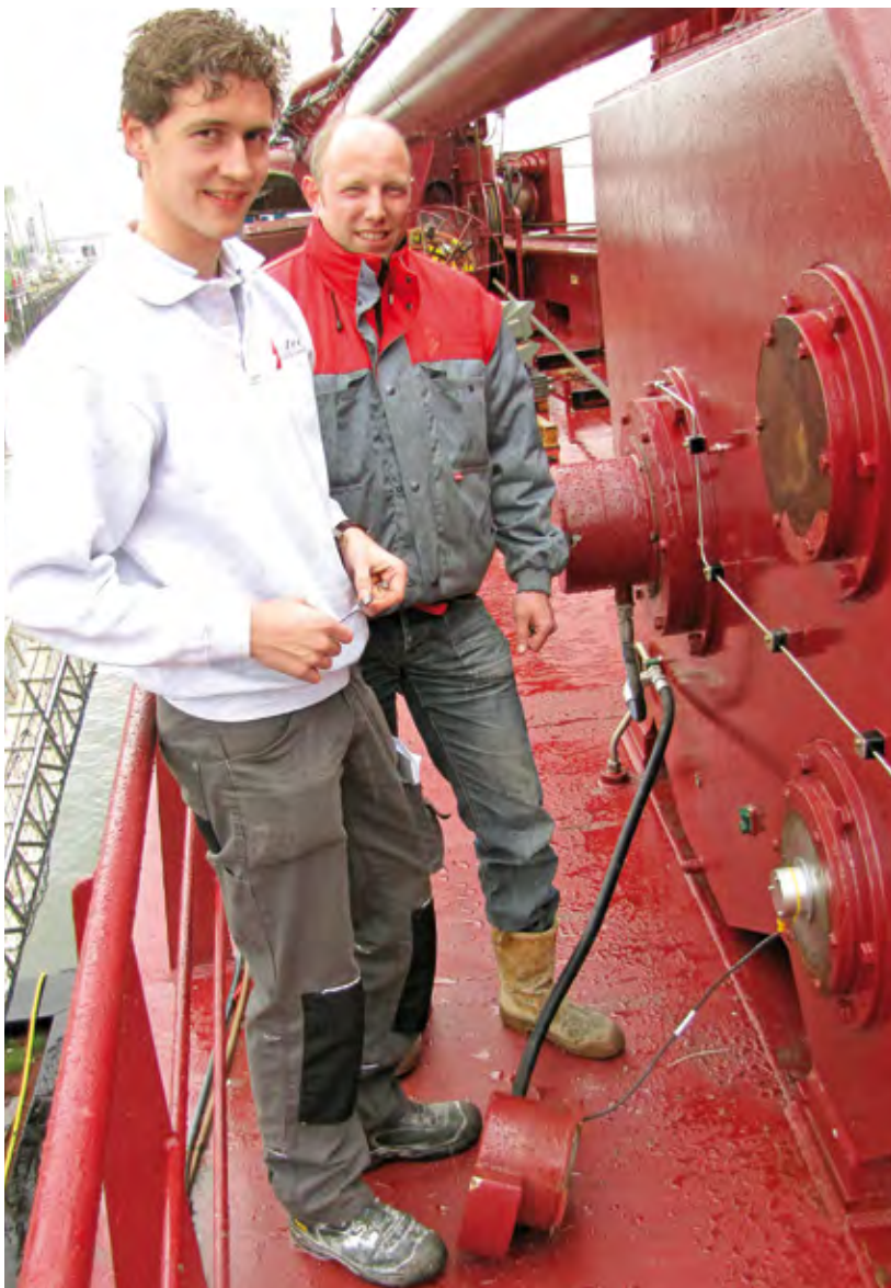
Sander Lensen and Dick de Vries (right) have removed the protective cover on the winch
