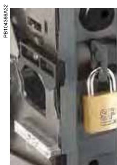
"Disconnected" position locking by padlocks.
